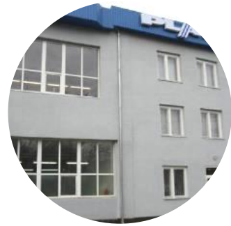
Foundation of production site in Vinogradiv, Ukraine (PLATI Ukraine Limited)
